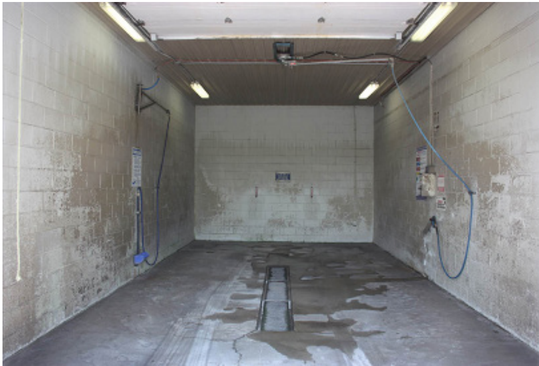
Compliments of Davis Duels, Burford, ON Scum precipitation build-up on the walls and floors Applied: TCI 303 H.D. Powerwash at 2,000 psi bottom to top Walls and floors received no other treatment e.g. paint.
