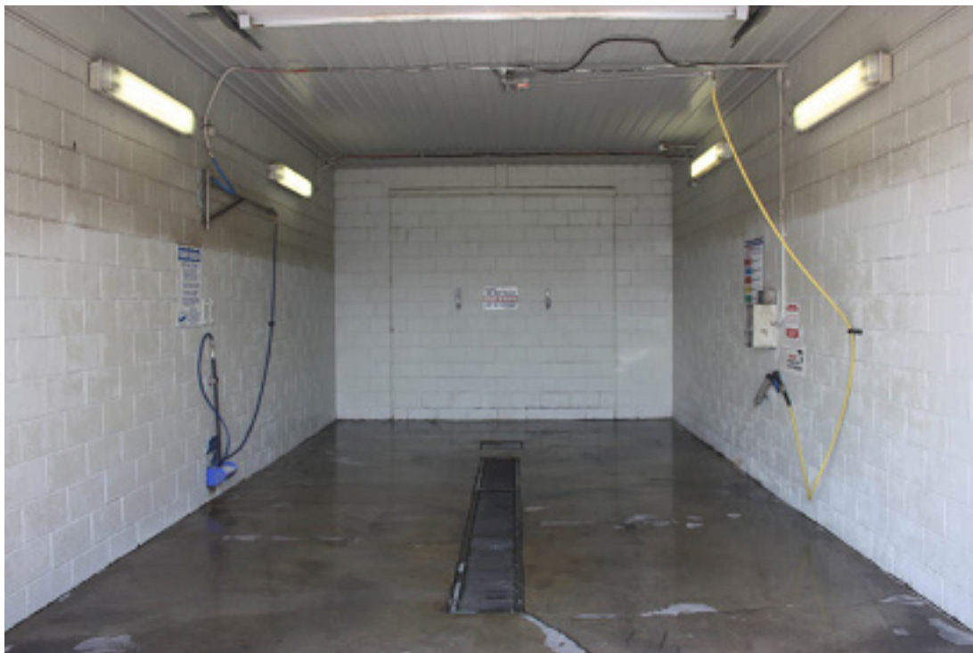
Compliments of Davis Duels, Burford, ON Scum precipitation build-up on the walls and floors Applied: TCI 303 H.D. Powerwash at 2,000 psi bottom to top Walls and floors received no other treatment e.g. paint.
