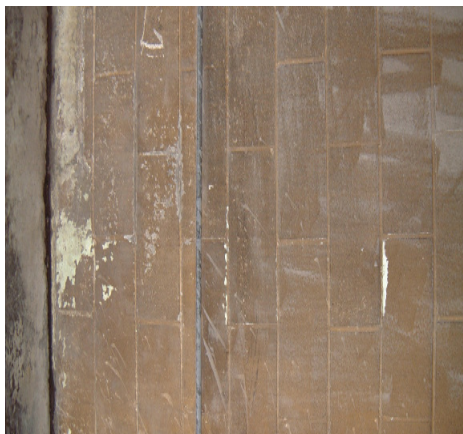
Block wall — before
